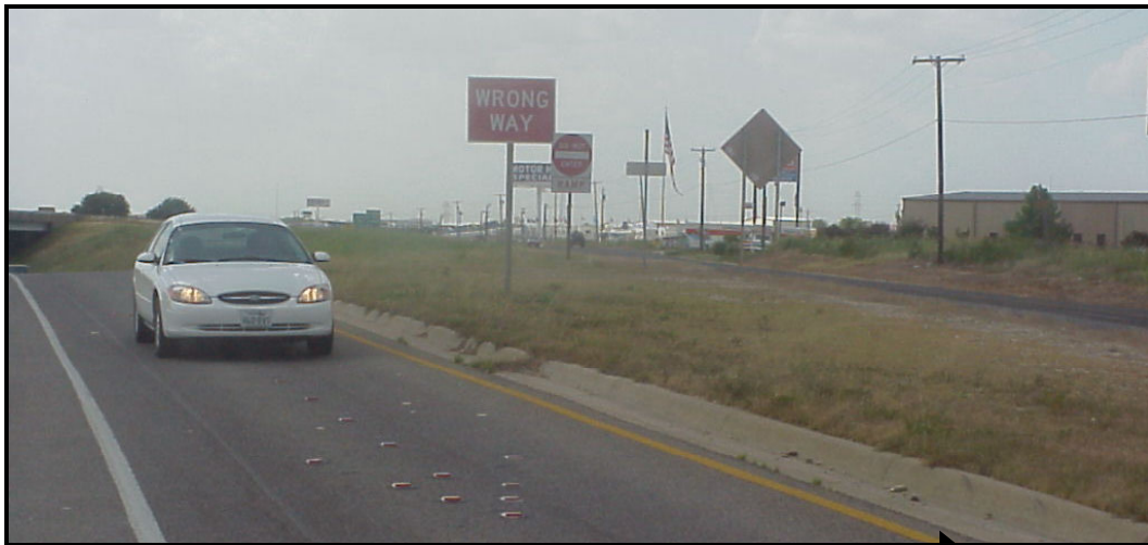
Figure 21. Example of Yellow Edge Line Wrong-Way Countermeasure.
