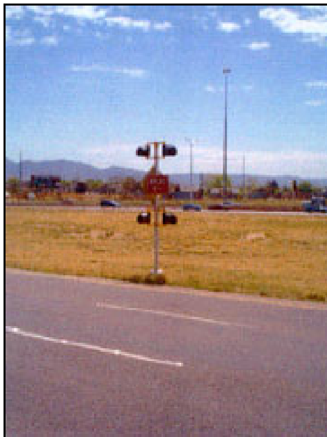
Figure 33. Picture of the New Mexico Directional Traffic Sensor System.
