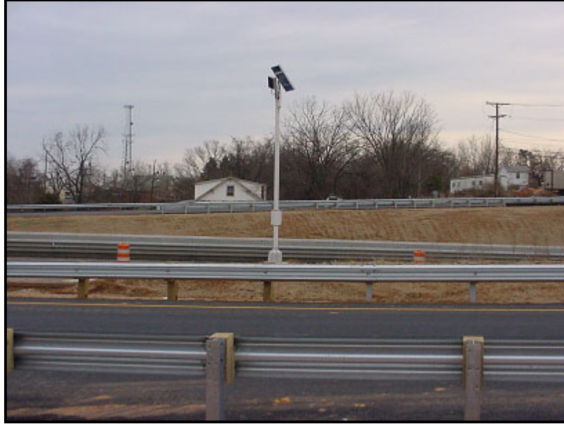
Figure 36. SAS-1 Acoustic Detector Installed on an Exit Ramp.
