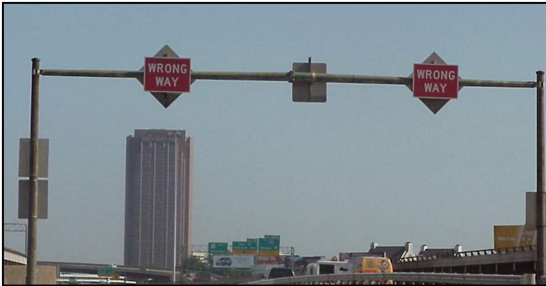
Figure 30. Overhead-Mounted WRONG WAY Signs in Texas.
