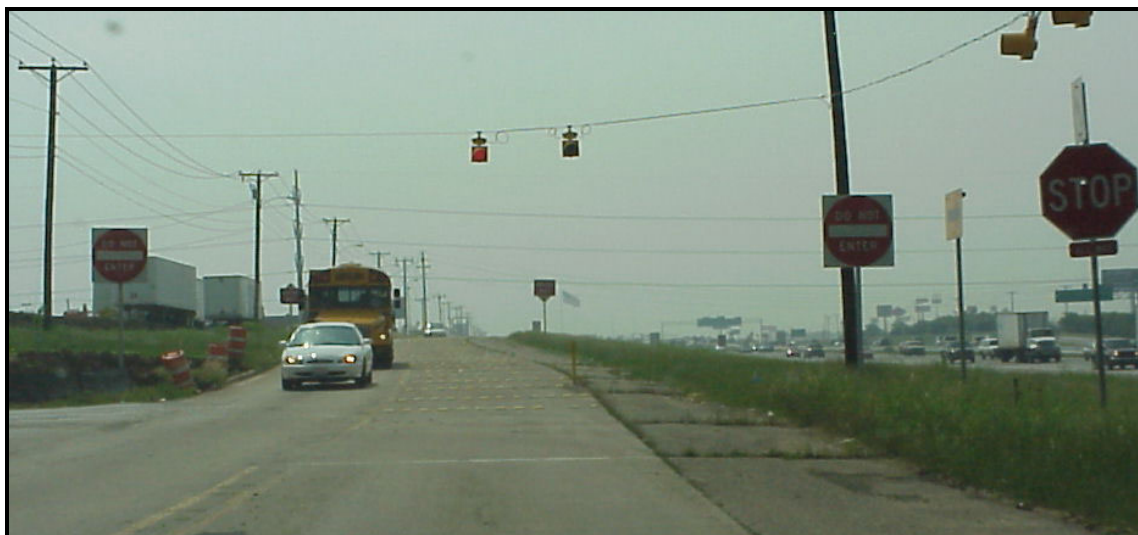
Figure 31. Overhead-Mounted Red Flashers on Span Wire in Texas.
