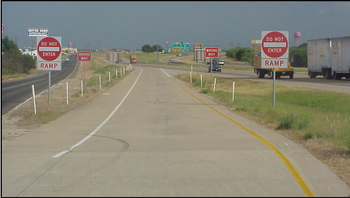
Figure 24. DO NOT ENTER Signs with RAMP Supplemental Placards.
