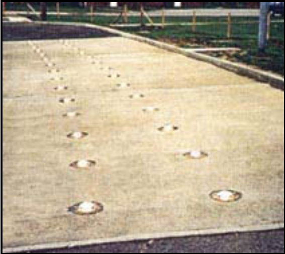
Figure 38. In-Pavement Warning Lights for Wrong-Way Vehicles.
