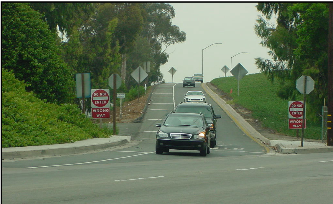
Figure 22. Lowered DO NOT ENTER/WRONG WAY Sign Package Used in California.
