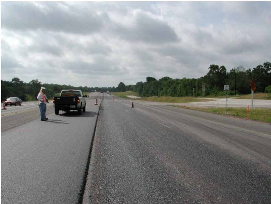
Figure 26. SH 6 Test Site Starting at RM 602.
