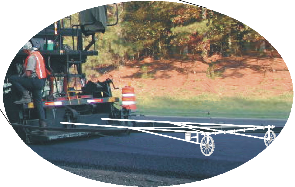
Figure 80. Concept Infrared Sensor Bar for Quality Control.
