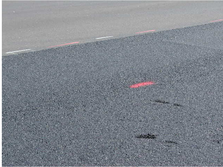
Figure 53. Close-up of Cold Streak Shown in Figure 52.
