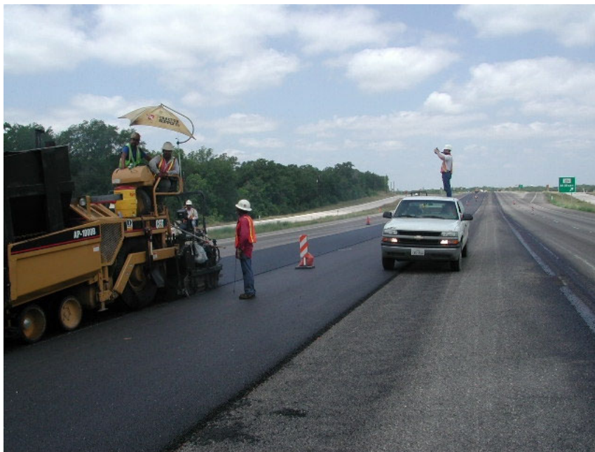
Figure 25. Infrared Imaging in Progress.
