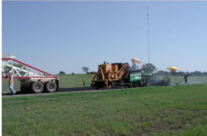
Figure 50. Paving Operation on IH 10 WB.
