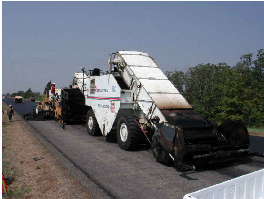
Figure 36. Paving Train on US 79.
