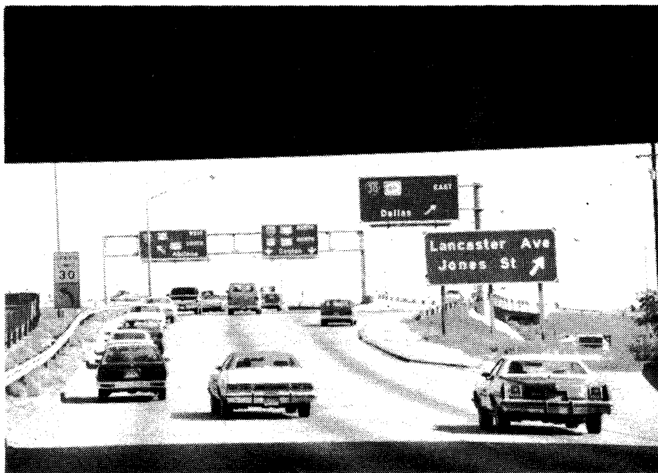
Figure 4-7. Lancaster Ave., Jones St. Exit Sign Location - Site 1 (300 Ft. From Gore Area).
