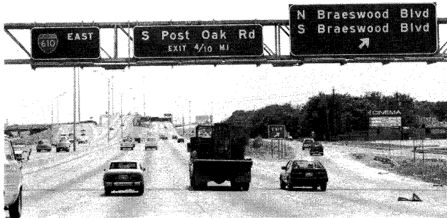
Figure 4-21. Braeswood Blvd. Exit Sign Location - Site 3 (2100 Ft. From Gore Area).
