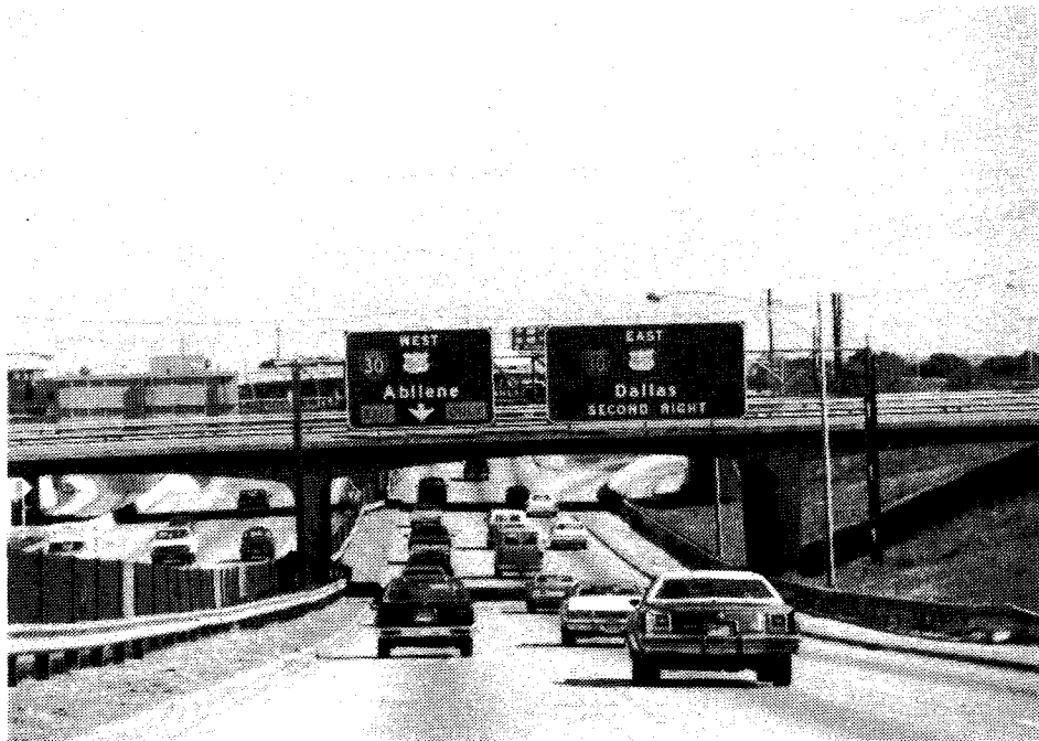
Figure 4-5. Vickery Blvd. Overpass Sign Location - Site 1 (1250 Ft. From Gore Area).
