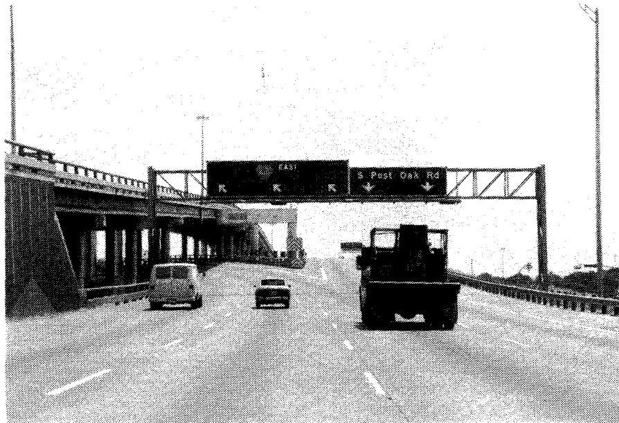
Figure 4-23. Gore Area Signs - Site 3.
