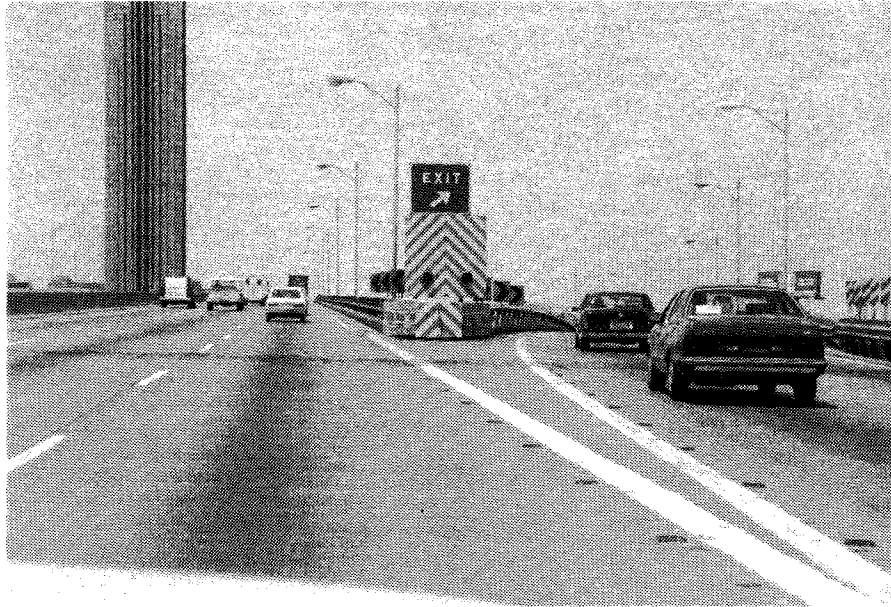
Figure 4-11. Crash Cushion And Pavement Delineation - Site 2 (Houston).
