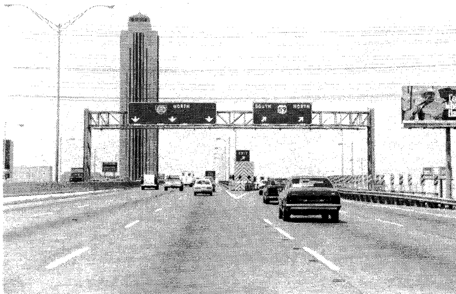
Figure 4-16. Gore Area Signs - Site 2.
