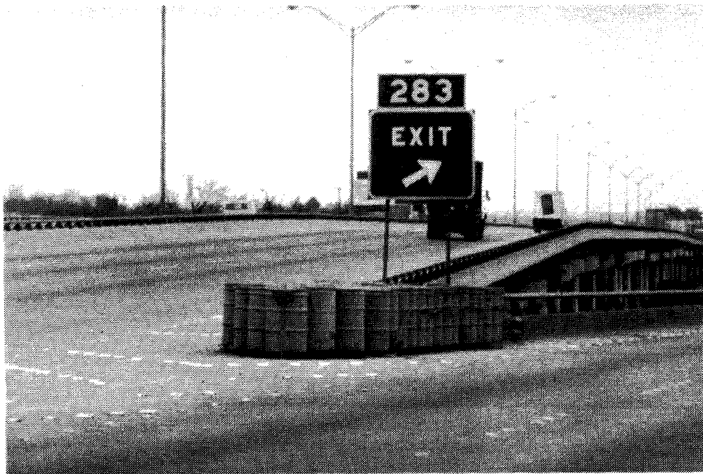
Figure 2-2. Chevron Nose Panel and Type 1 Object Marker At Front of Crash Cushion.
