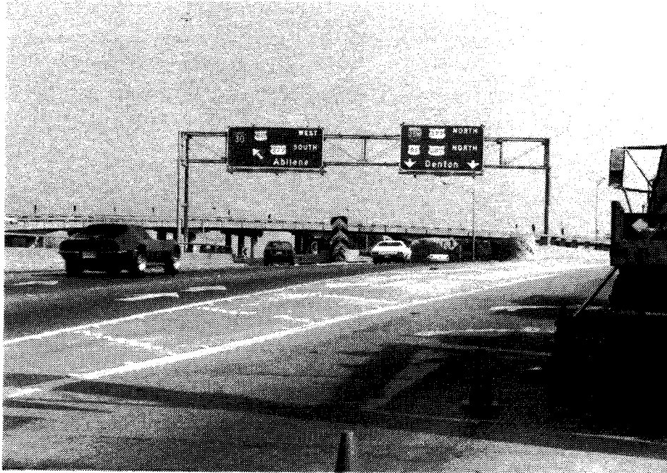
Figure 4-3. Crash Cushion and Pavement Delineation - Site 1 (Ft. Worth).
