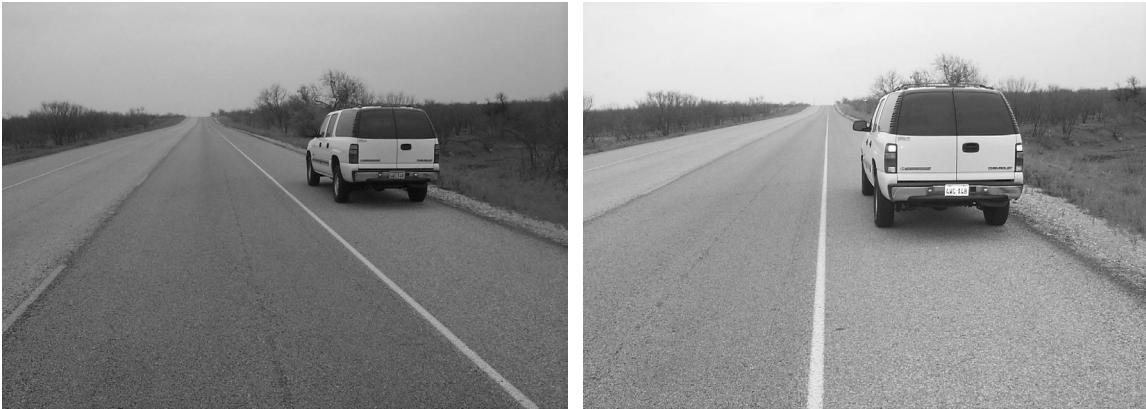
Figure 17. Photograph for Question 11, 10-Ft Shoulder.
