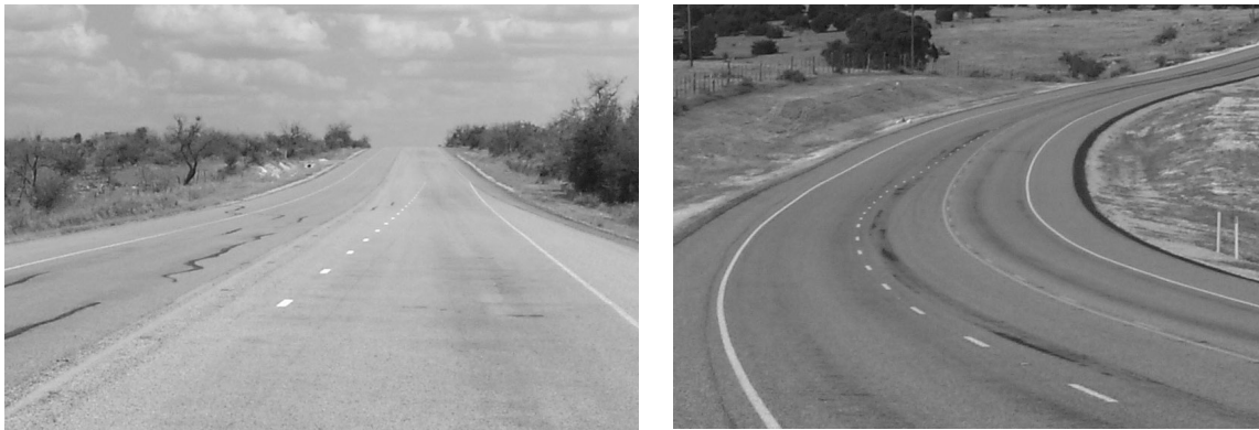
Figure 50. Texas “After” Passing Lane Entrance Markings.
