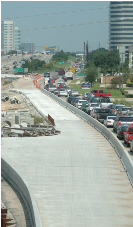
Construction of toll road ramp
