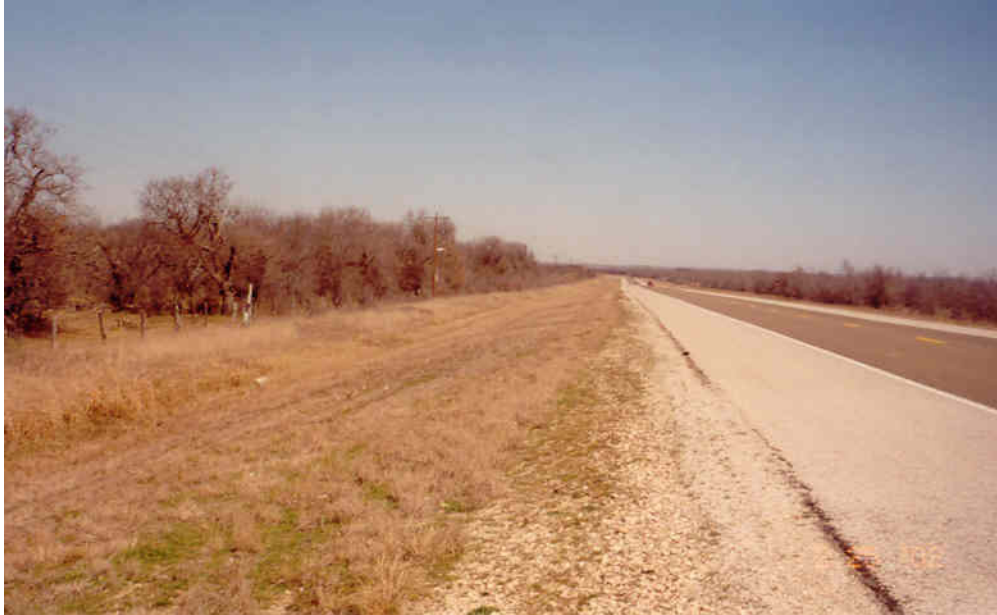
Figure 6. Photograph of a Potential Site for an Installation of an Animal Crash Countermeasure.
