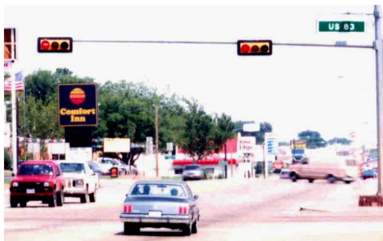
Figure 13. Strobes in Signal Heads.
