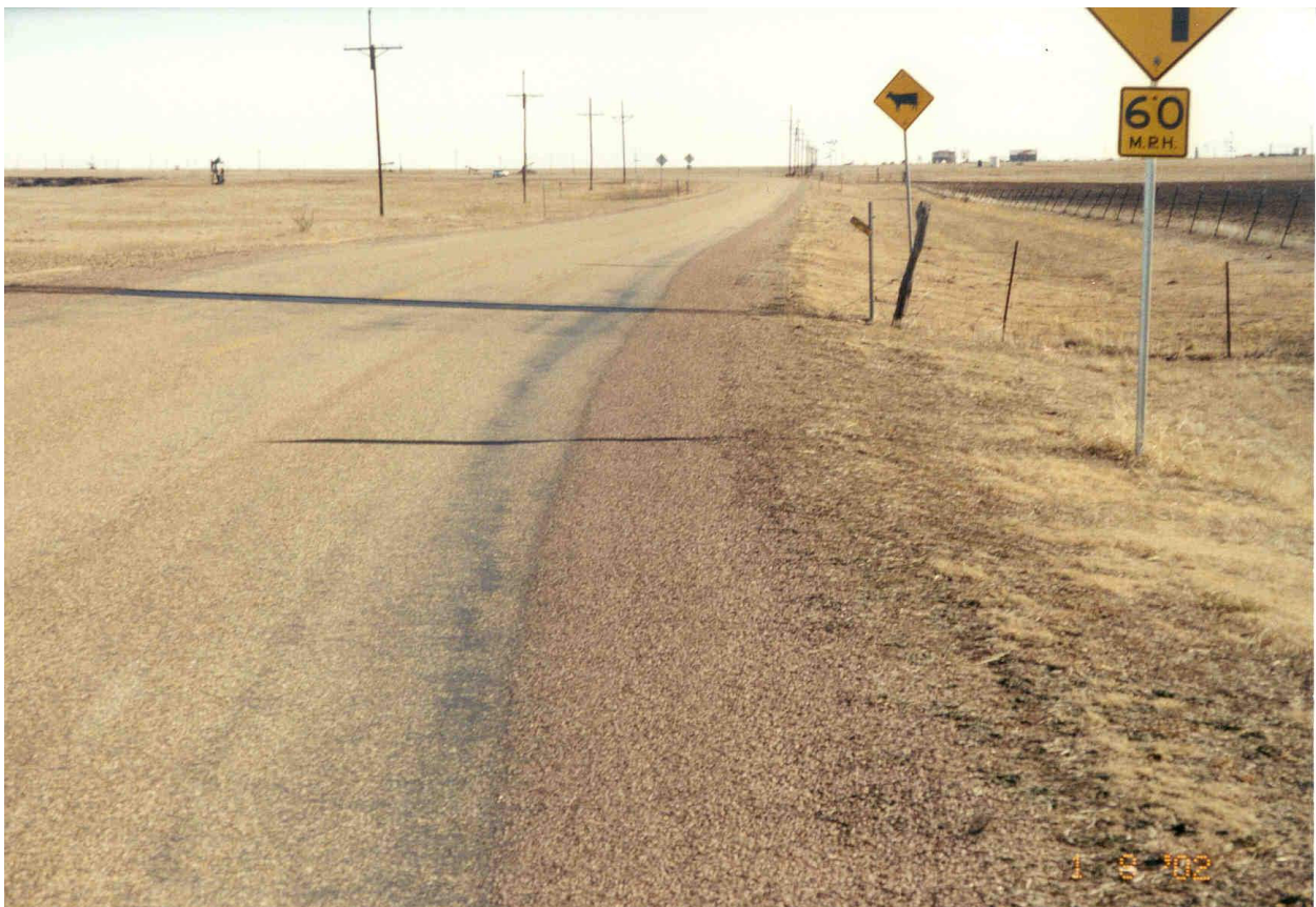
Figure 16. View of Comparison Site near Site with Roadway Widening.
