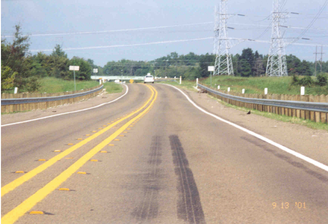
Figure 11. View of Added Raised Pavement Markers and Delineation.
