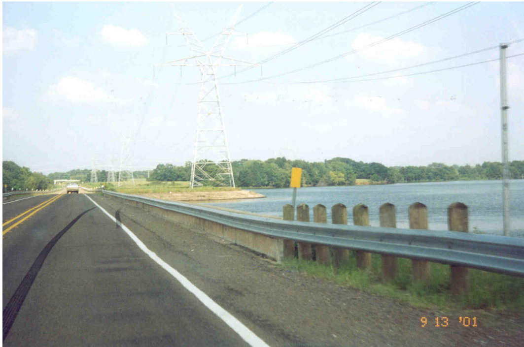
Figure 10. View of Bridge on Lake.
