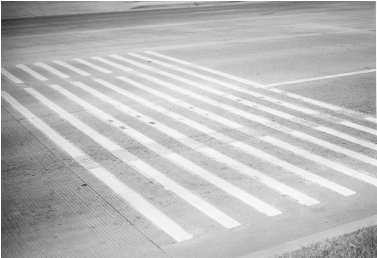
Figure 14. Close-Up View of Approach Rumble Strips.
