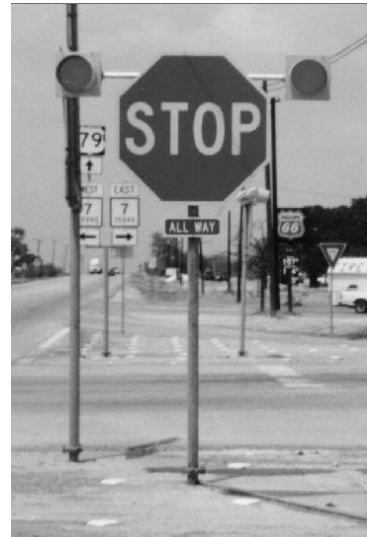
Figure G-5. Beacons on Stop Sign (9).
