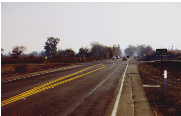
Figure G-1. Example of Left-Turn Lane (9).
