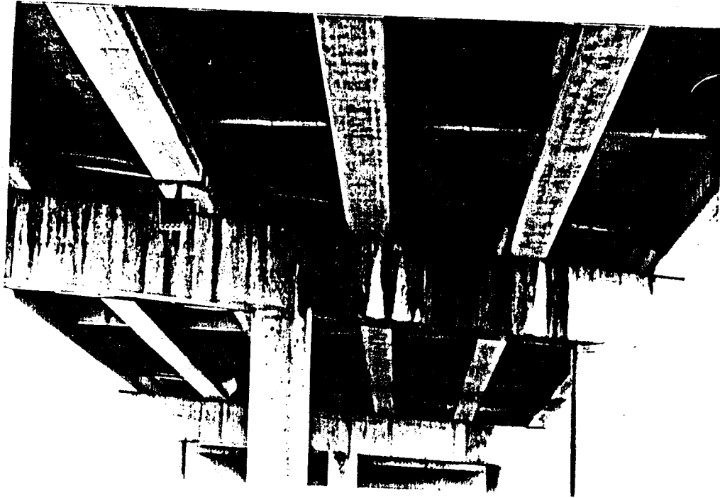
Figure 21. Deck runoff stains.
