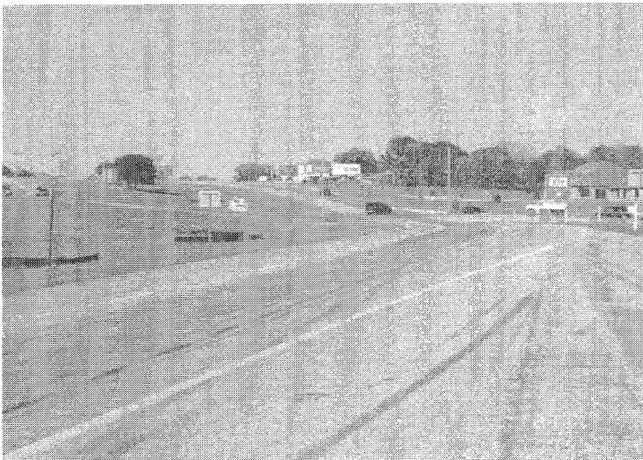
Figure A-4. U.S. 290 Westbound at F.M. 577, 500 ft from the Stop Line.
