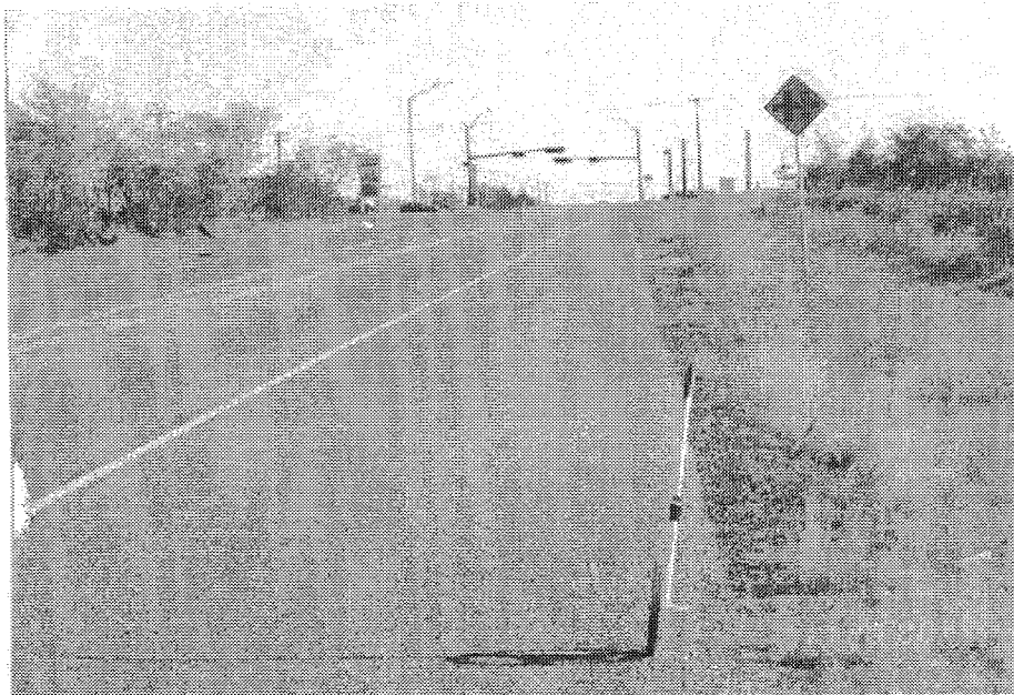
Figure A-12. F.M. 2154 Southbound at Rock Prairie Road, 1000 ft from the Stop Line.
