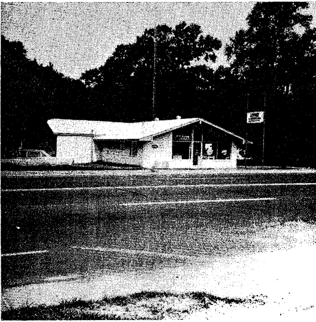
Heating and Airconditioning
