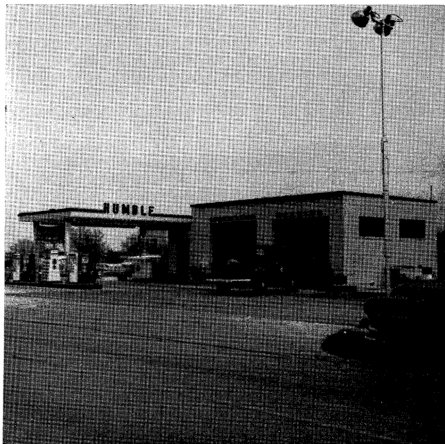
One of the newer service stations located along the old route.
