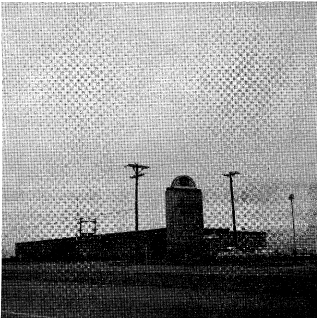
Plenty of room for building and parking sites are also important.
