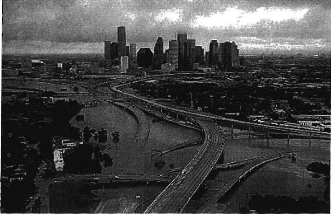
Figure 24. Tropical Storm Allison Flooding.
