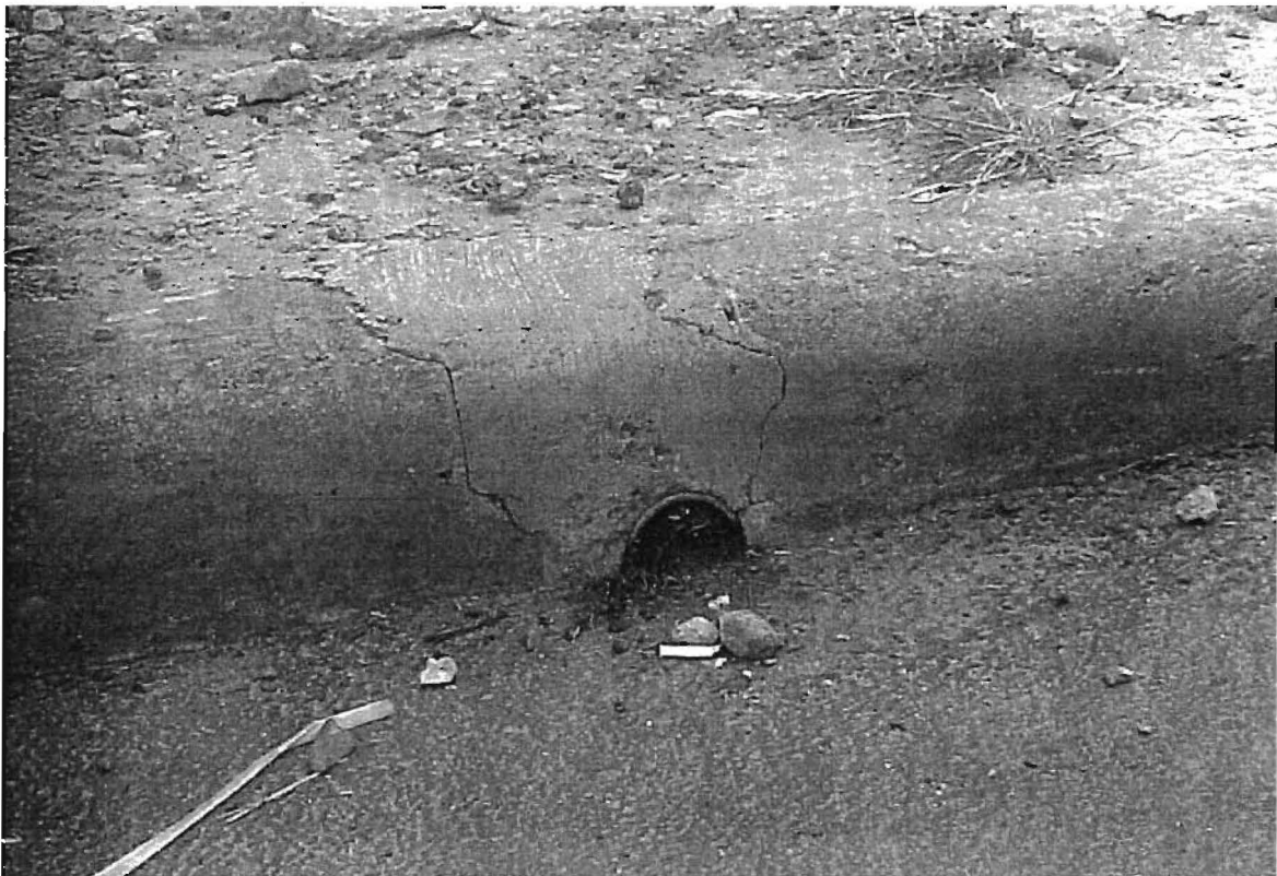
Figure 12. Curb-Mounted Roadway Water Depth Pressure Transducer.
