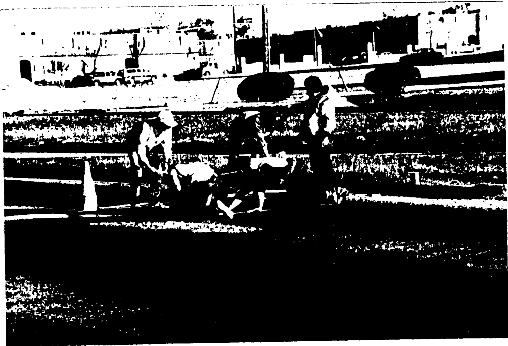
Placing Loop in Inner Lane.
