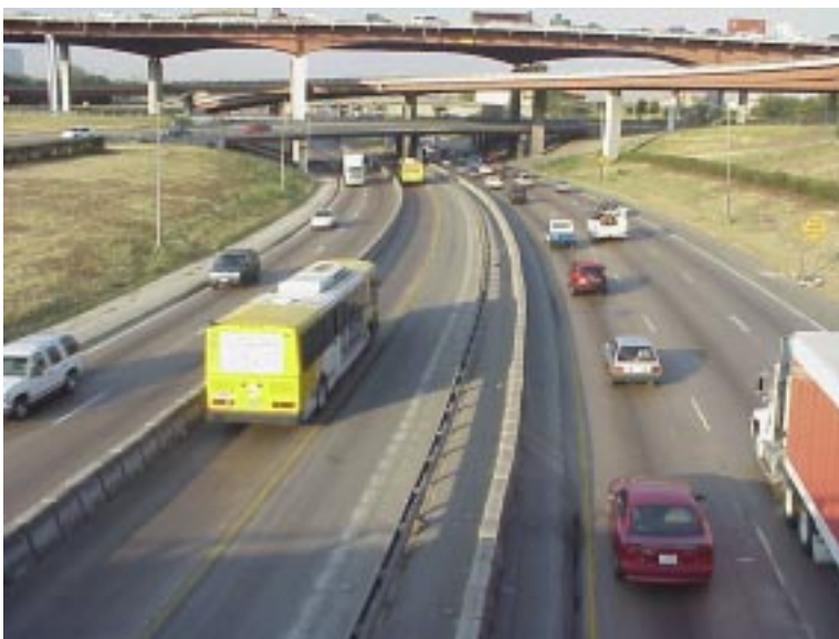
Figure 1. Barrier-separated contraflow lane
