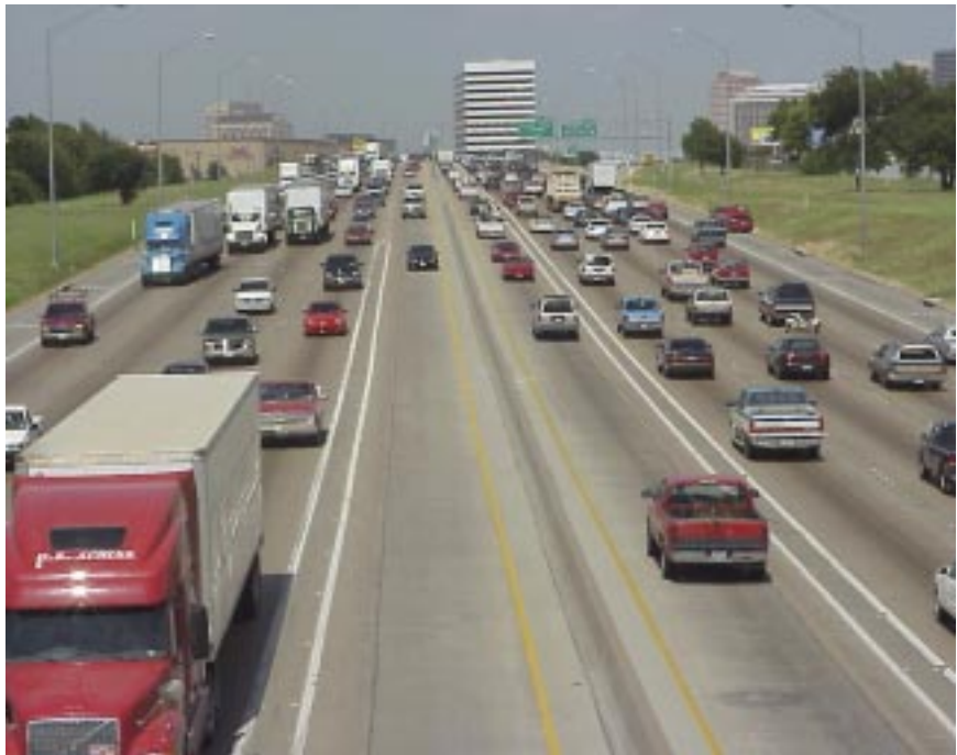
Figure 2. Buffer-separated concurrent flow lanes
