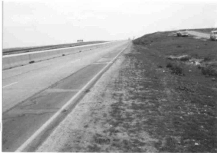
Figure 12. Water Accumulating on the Concrete-Asphalt Interface.
