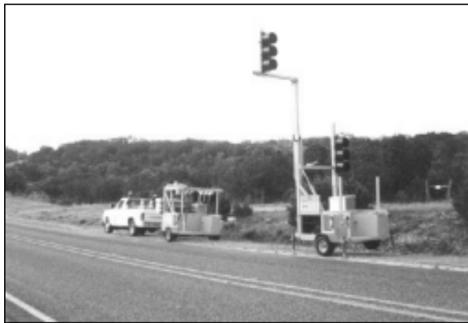
Figure 1. Field Setup of Portable Traffic Signals.
