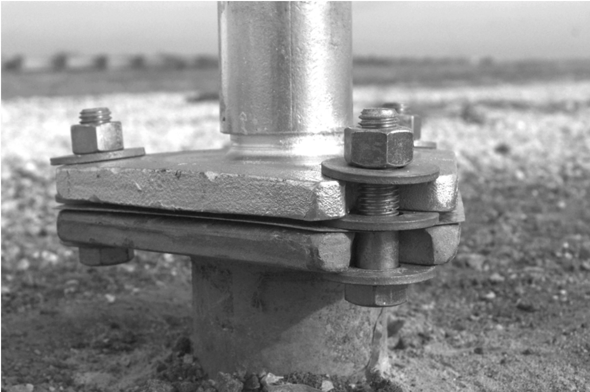
Figure 4. Sign Support Installation before Test 439117-3.
