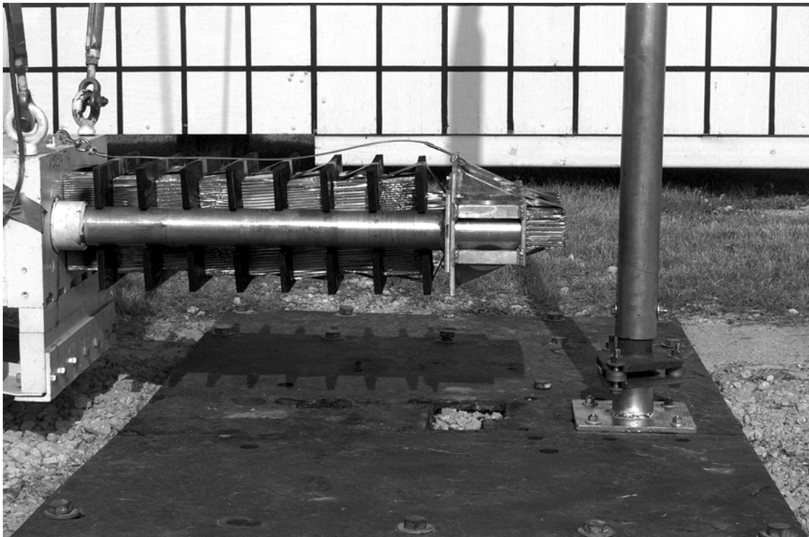
Figure 19. Typical Sign Support Installation before Pendulum Testing of Lifting Cone.
