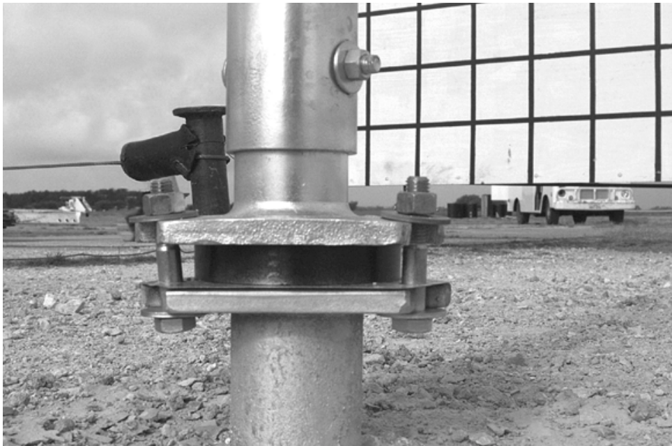
Figure 21. Installation before Test 439117-1.
