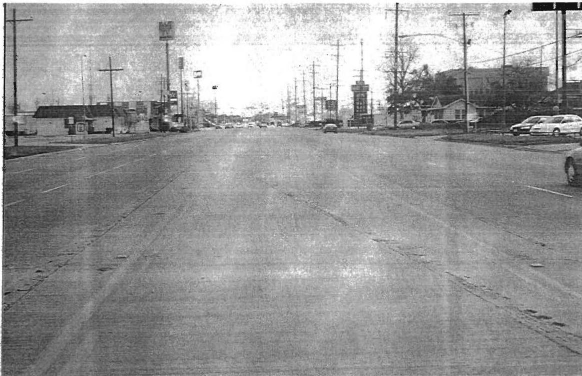
Figure 15. Southbound Twin Cities Highway North of Texas 73
