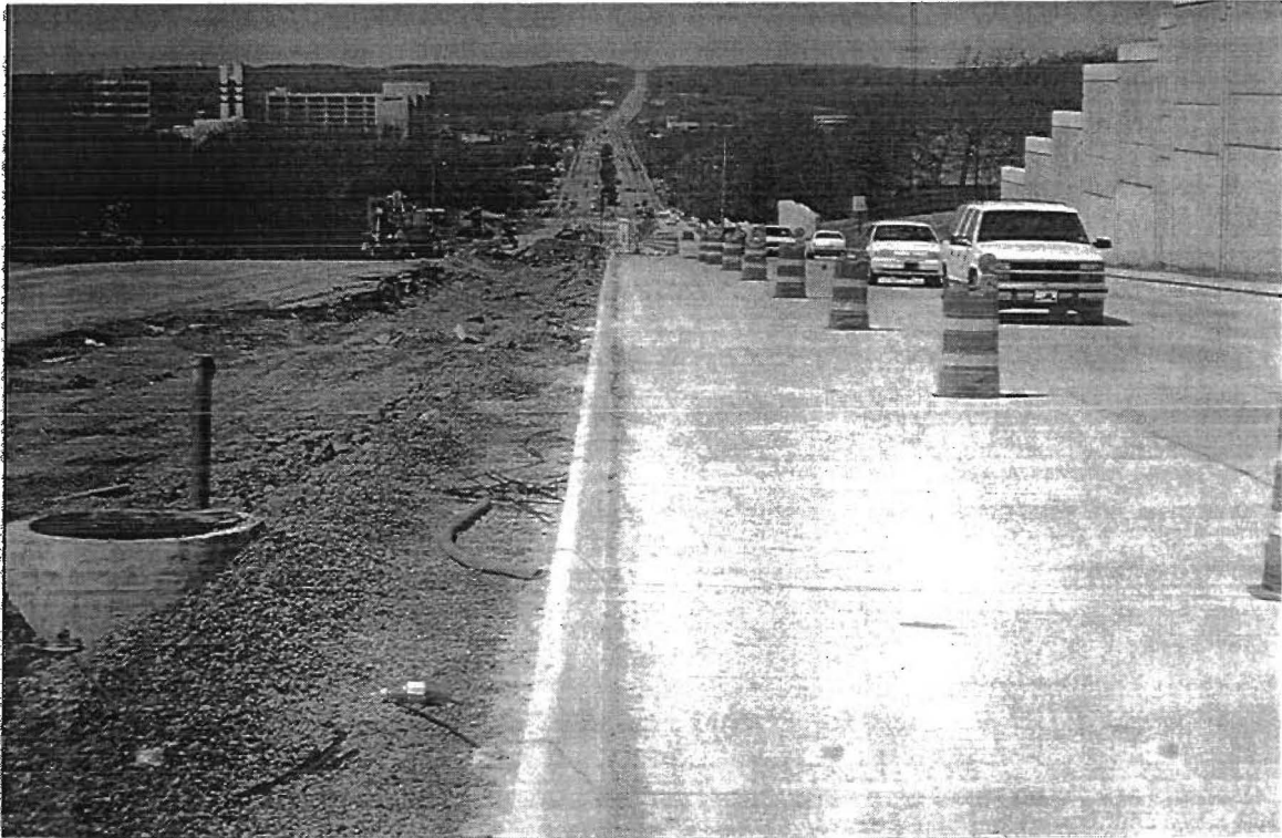
Figure 33. Westbound 71 st Street West of Harvard Avenue
