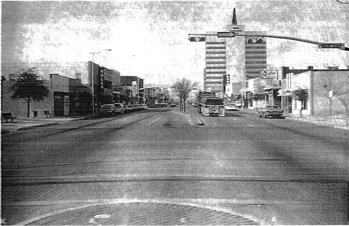
Figure 29. Northbound Grant Avenue at 4 th Street
