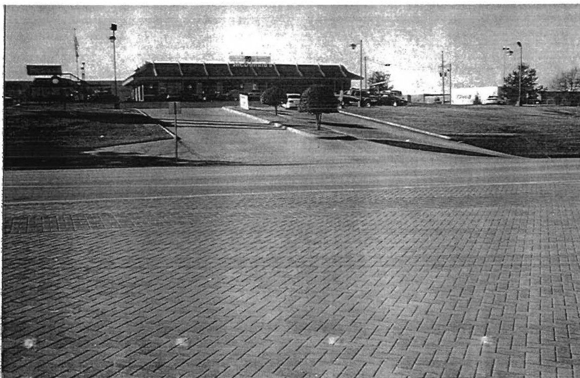
Figure 24. Facing South on Loop 281 West of Tuttle Road
