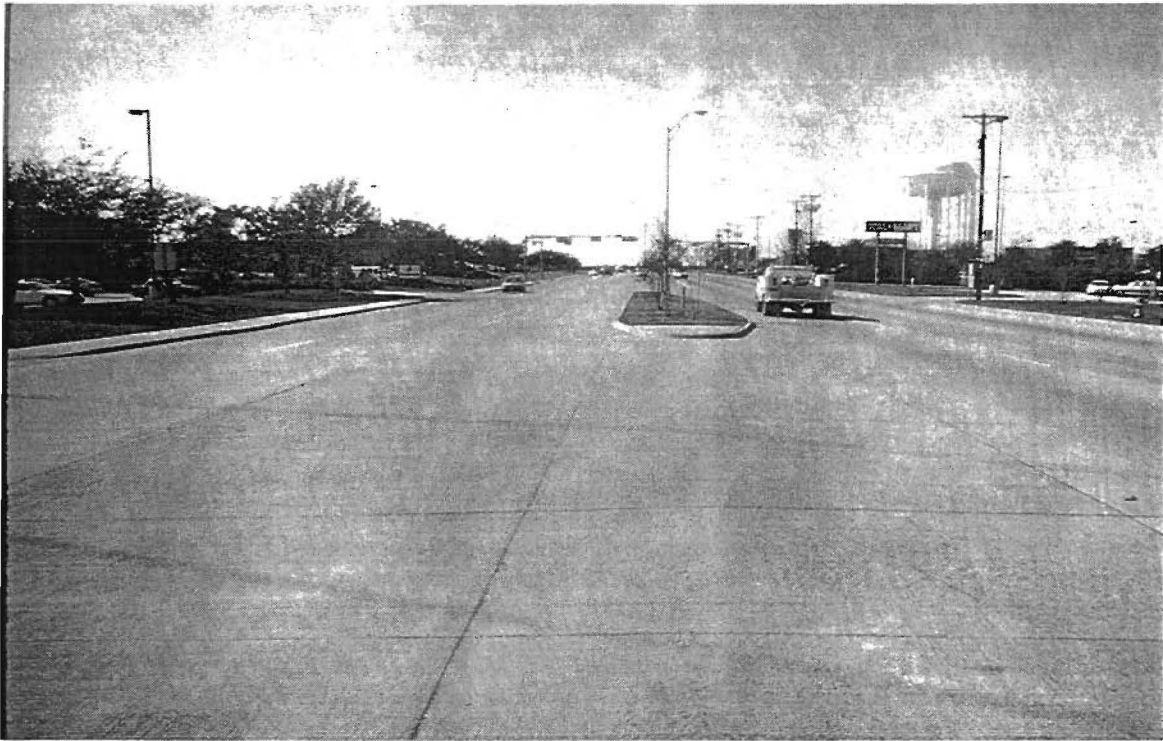
Figure 21. Westbound University Drive Near Graves Street
