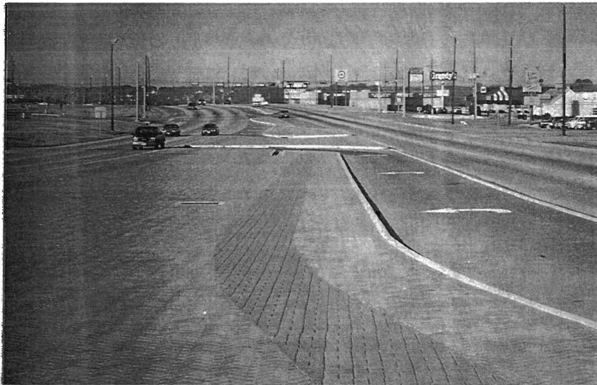
Figure 23. Westbound Loop 281 Between Judson Road and Tuttle Road
