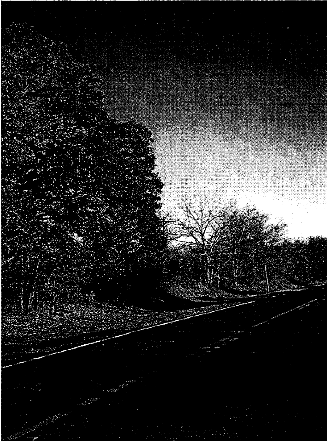
Figure 40. Large Trees Adjacent to the Cracked Section.
