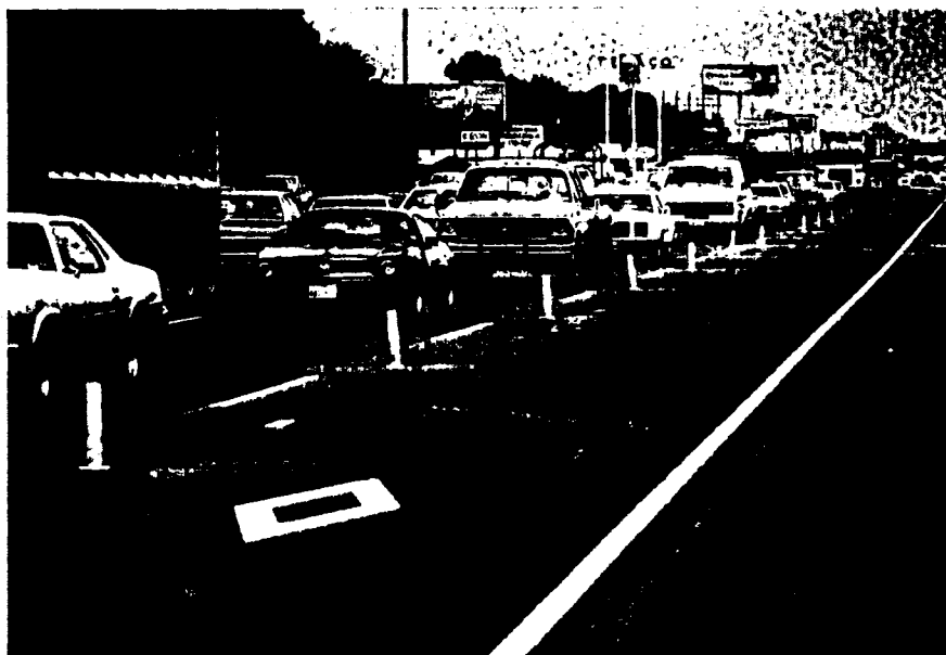
Figure 10. Contraflow Diamond Pavement Markings and Yellow Plastic Pylons
