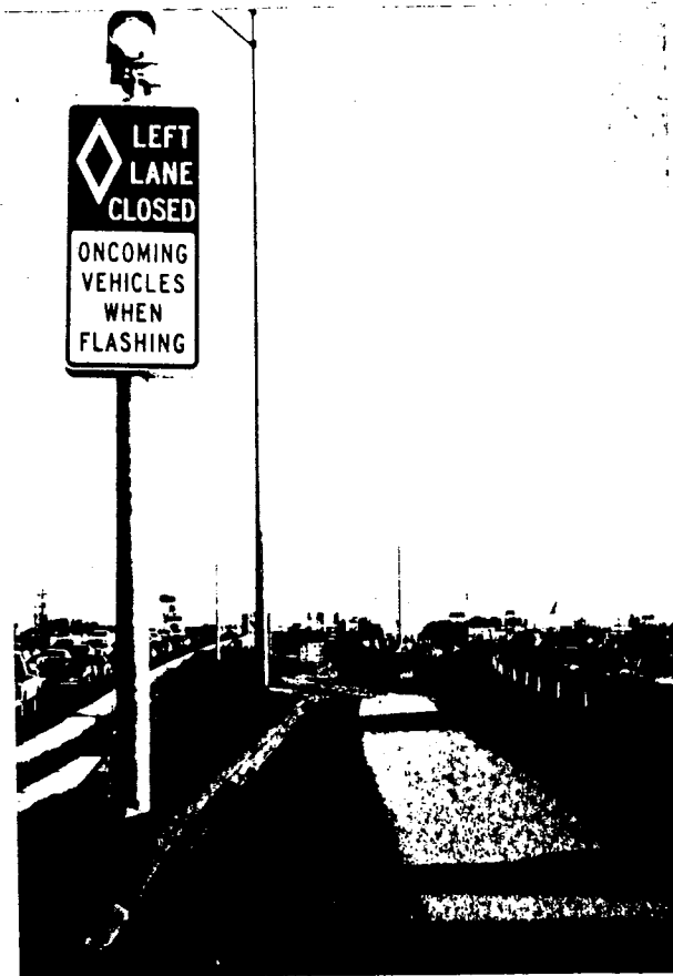
Figure 8. CFL Stationary Signs with Flashing Yellow Beacons
