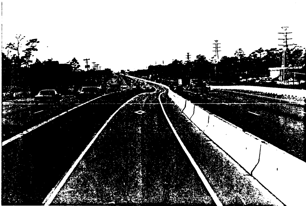
Figure 5. Katy Freeway Transitway Implementation: Curved Section
