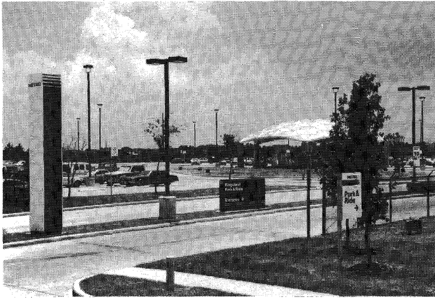
Figure 8. Kingsland Park-and-Ride Lot, Katy Freeway Corridor
