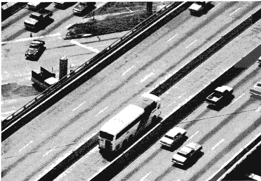
Figure 2-4. Elevated Transitway Mainlane Configuration
