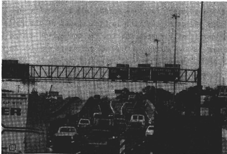
Figure 8. Advanced Signing for Bridge Deck Overlay Traffic Control
