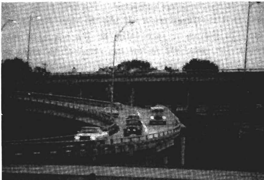
Figure 29. Vanpool Using I-45 North Transitway "Ramp.B"
