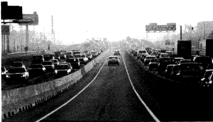
Figure 3: Straight Section of Katy Transitway
