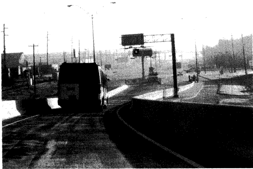
Figure 8: Elevated Flyover at Post Oak Terminal
