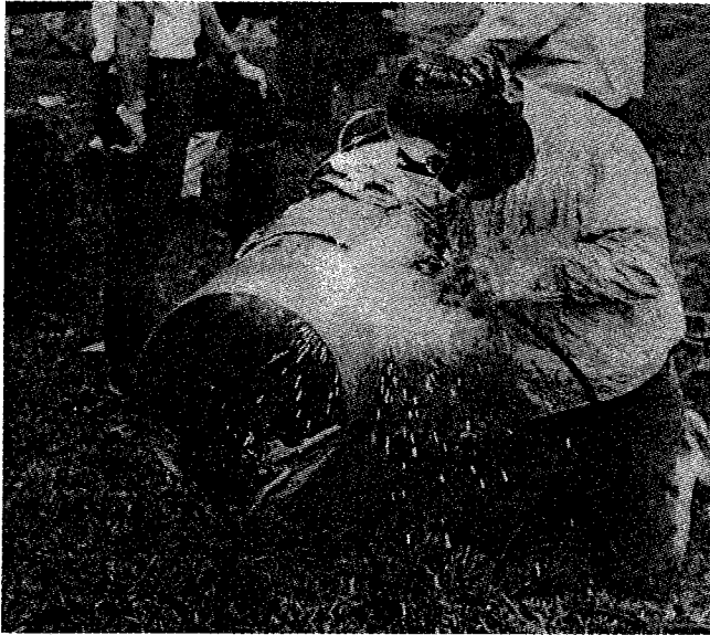
Figure 5.3. Welding open end segment.
