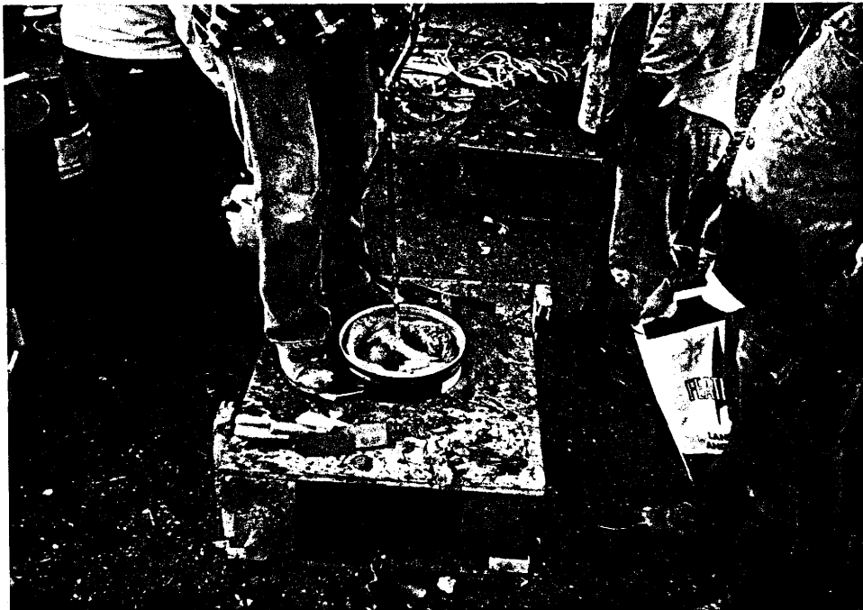
Figure 14. Mixing the Epoxy Mortar.
