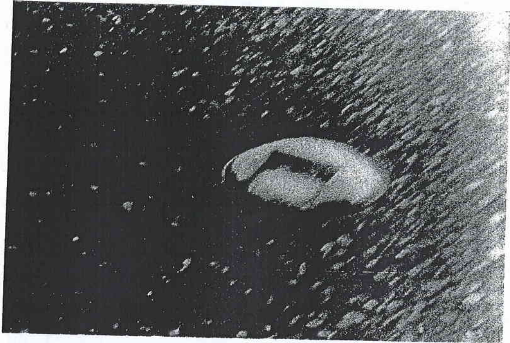
Figure 15. A RTB Submerged Into the Asphalt Pavement.
