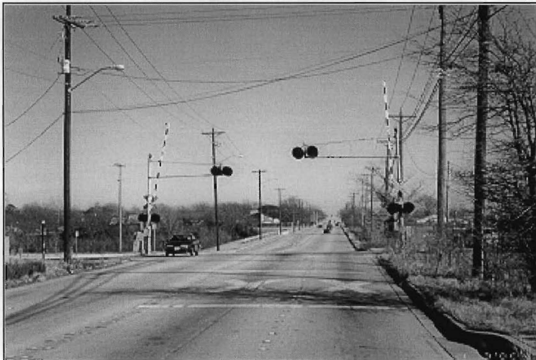
Figure 6-18. Photograph of Sycamore School Road.
