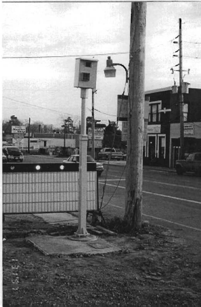
Figure 7-7. Photograph of Equipment at FM 2100 Site.
