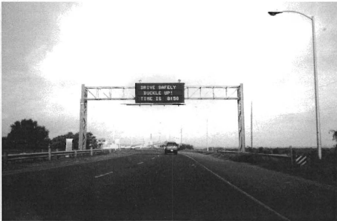
Figure 4.2 Existing Changeable Message Sign on South Padre Island
