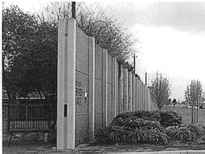
Figure 1. Typical Texas Soundwall
