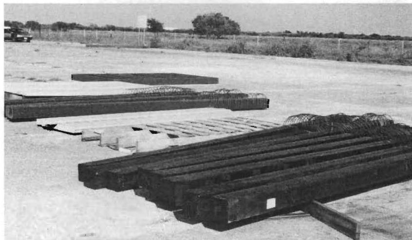
Figure 7. Materials Assembled to Construct Full-Scale Soundwall
