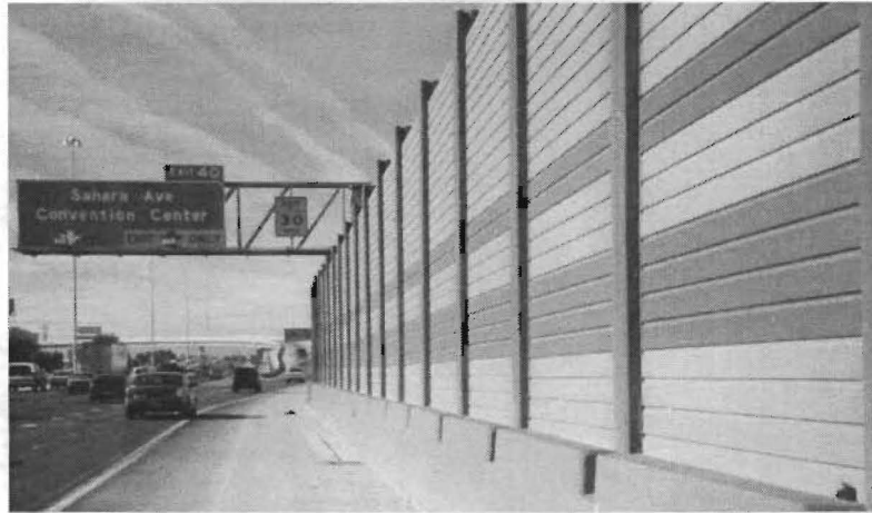
Figure 5. Conventional Soundwall Incorporating Plastic Materials
