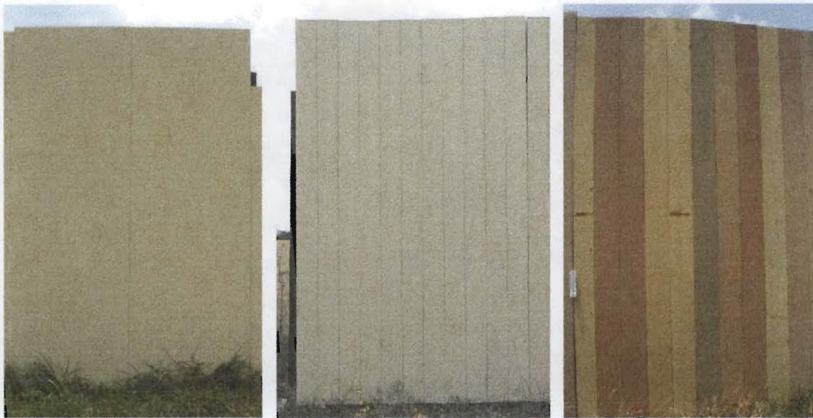
Figure 21. Modules: (a) Tan Sheet Plastic; (b) Tan Plastic Lumber; and (c) Multicolored Plastic Lumber
