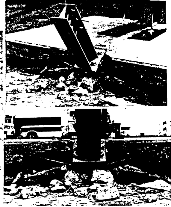
Deck Cracking in T101 Deck After Dynamic Test
