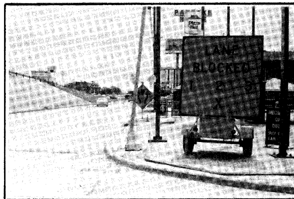
Figure 6-2. Advance Sign During Frontage Road Studies
