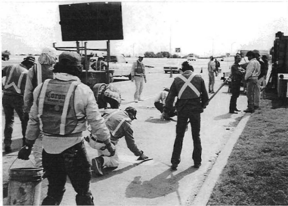
Fig. 4.3. Placing of Repair Mixture.
