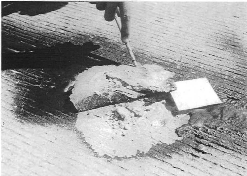
Fig. 3.13. Repair No.16 with Flamecoat PH101 Observed on October 20, 1993.
