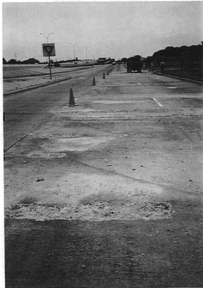
Fig. 4.2. A View of the Repair Section After the Spalls Were Cleaned.
