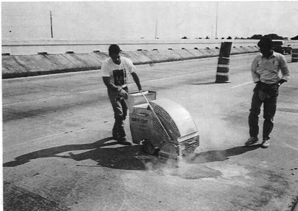
Fig. 4.4. Saw Cutting.
