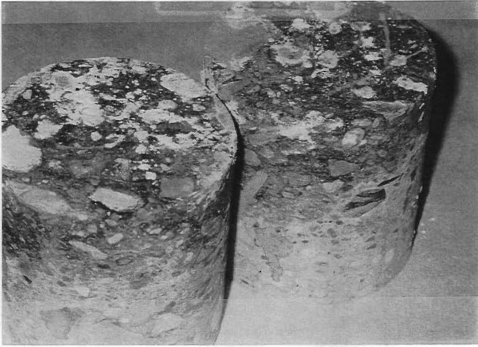
Figure 12. Signs of Efflorescence on Core Samples from SH 36.
