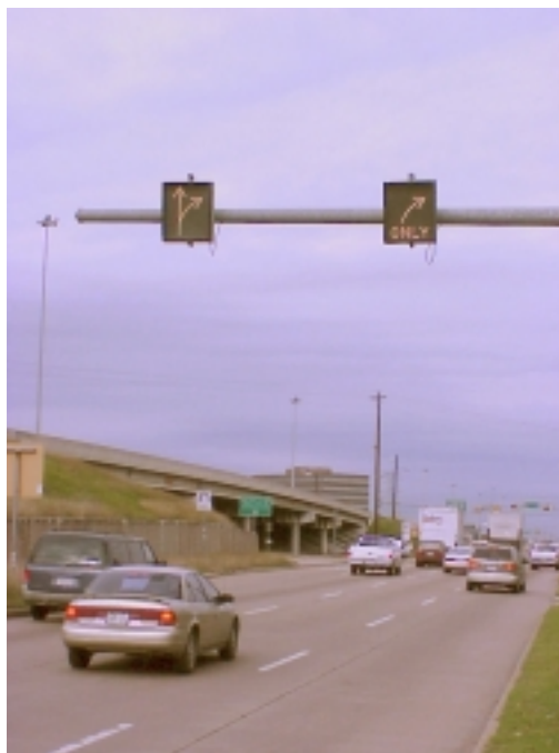
Changeable Lane Assignments Signs (CLAS) offer a potentially effective solution to changing traffic conditions
