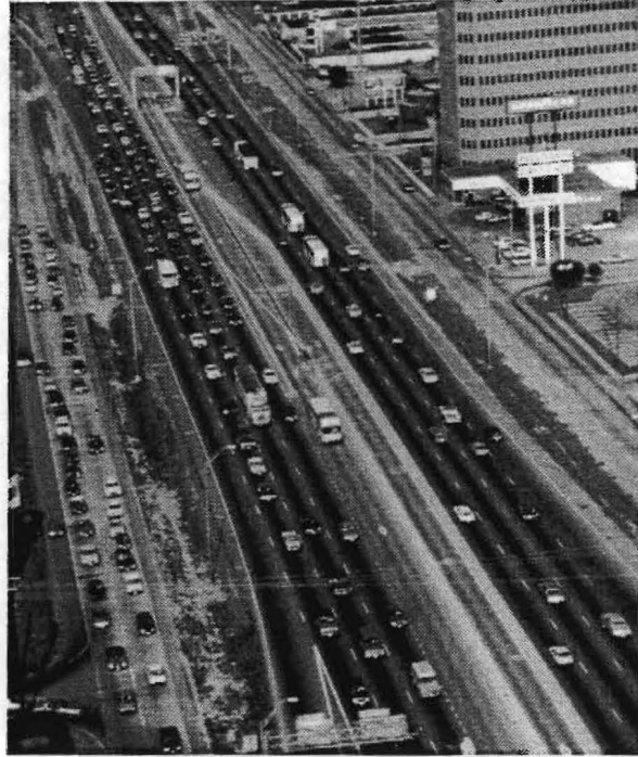
Figure 8. "Slip Ramp" Access Treatment
