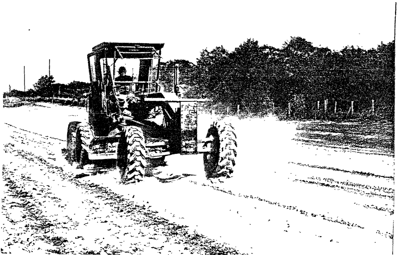
Figure D-5. Motor Patrol Initially Mixing Fly Ash with Soil.
