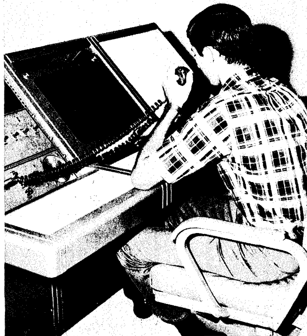
MONITOR ARRANGEMENT IN CENTRAL CONTROL CENTER
