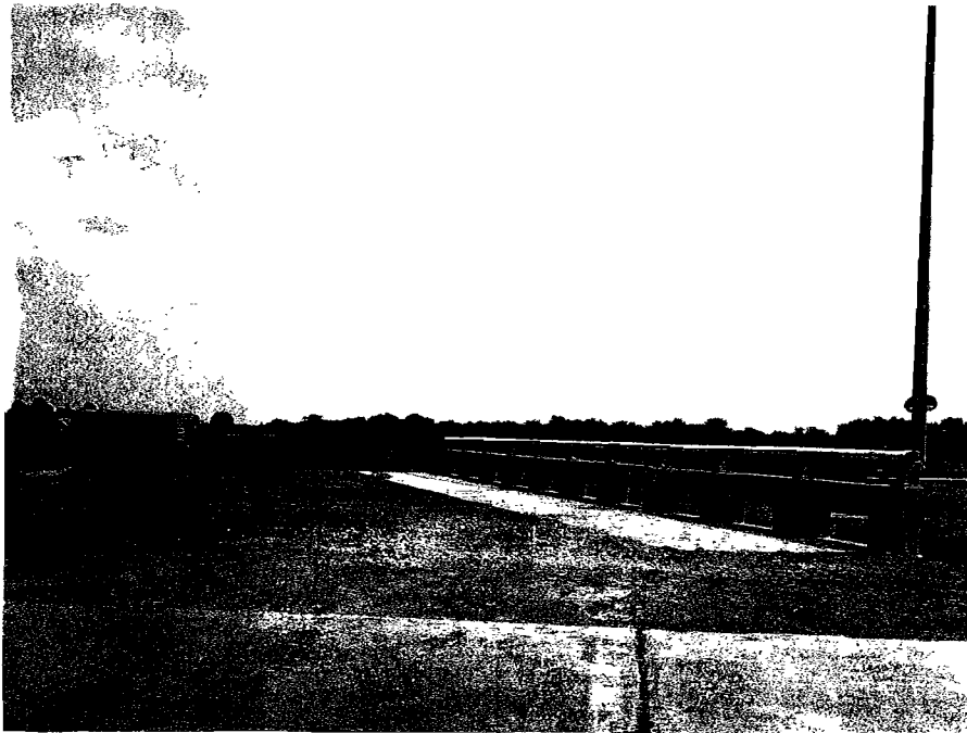
Figure 3. Front View Before and After Photographs of Bridge Rail for Test 3.
