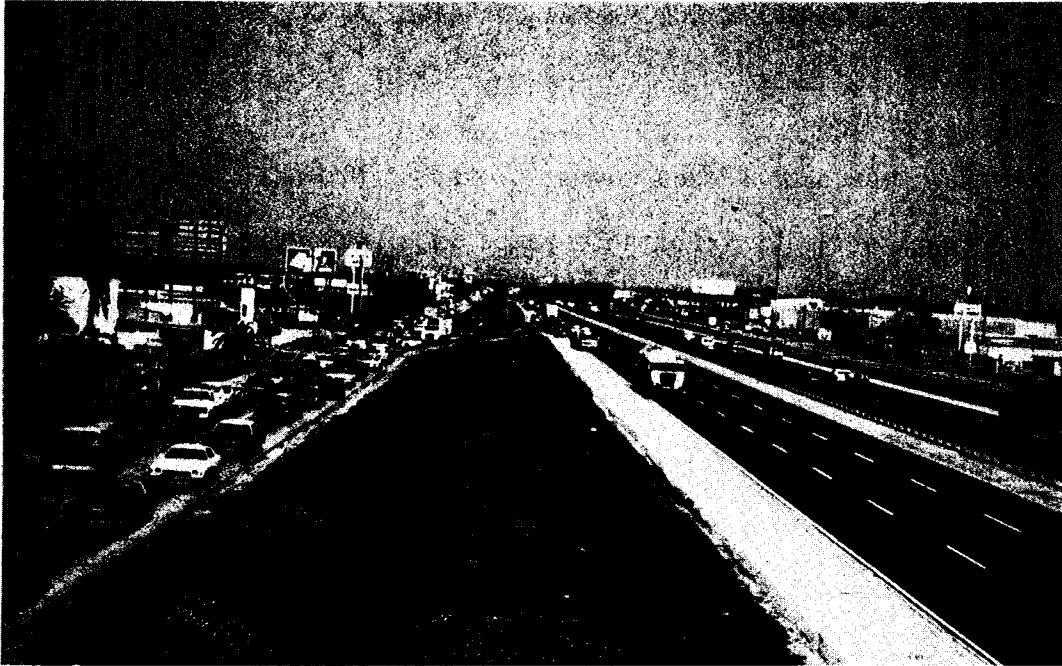
Figure 6a. Frontage Road Congestion at Freeway Work Zone Where Entrance Ramps Were Closed Too Soon
