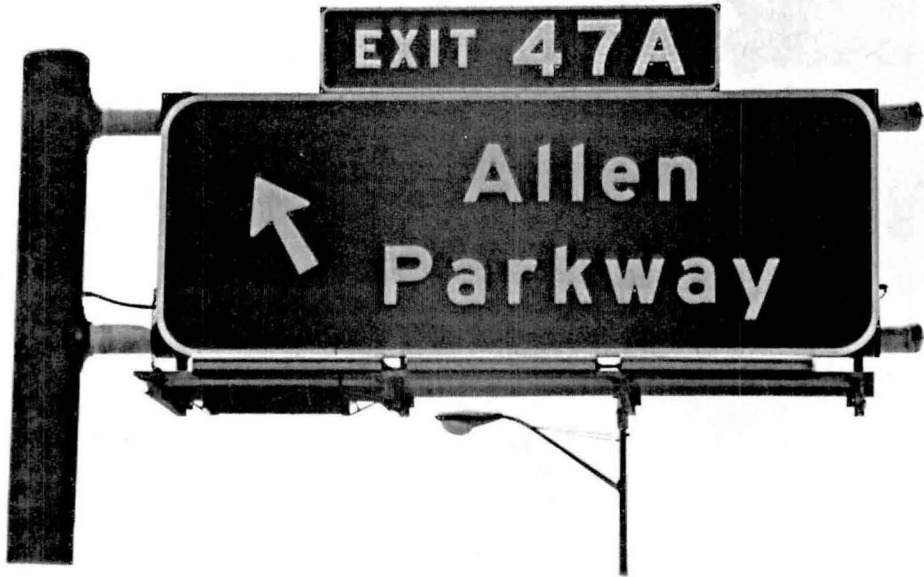
FIGURE 8. High Specific Intensity - High Specific Intensity Legend and Border - Initial Installation (Aluminum Sheet Overlay)
