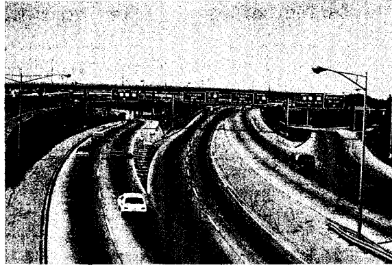
Figure 1-9. I-35E Junction With I-30 In Dallas.
