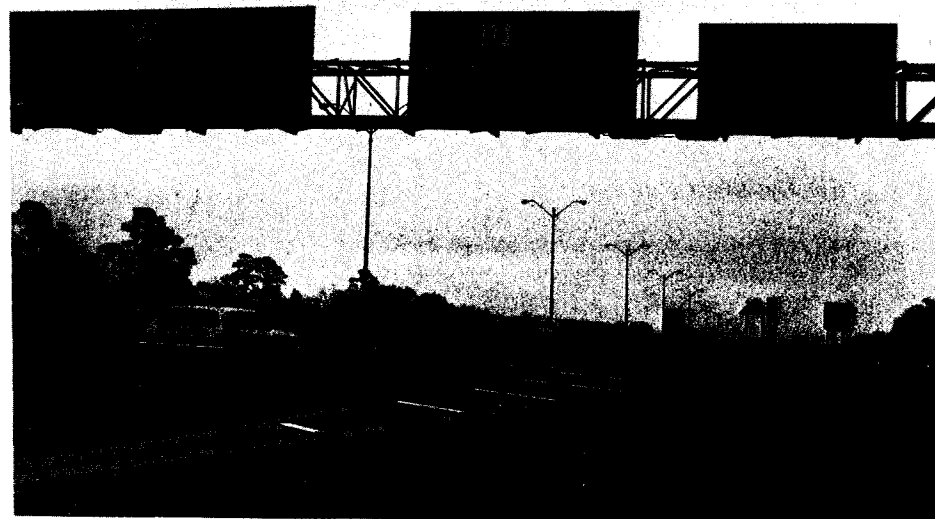
Figure 2-1. Sequence of Three Existing Overhead Sign Structures Along Section 'A' of I-10 in Houston.
