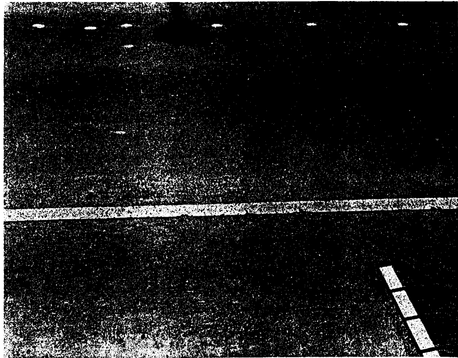
Figure 2.5. Outside Traffic Lane and Shoulder, Structure 98
