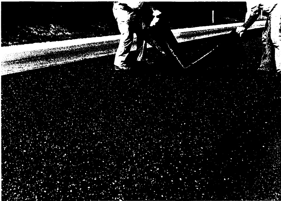
FIGURE 2: DETERMINATION OF AGGREGATE SPREAD QUANTITIES
