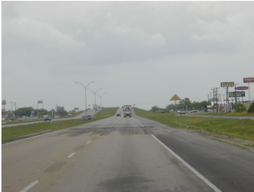
Figure 3-4. Site 2 – Photo of I-410 at Station 1 (San Antonio, Texas).
