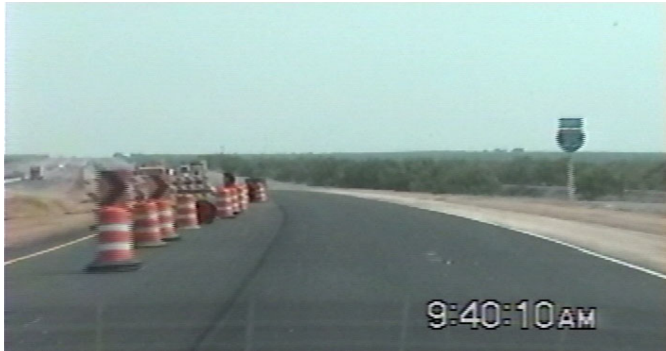
Figure 3-12. Site 3 Photo of Merge Area.
