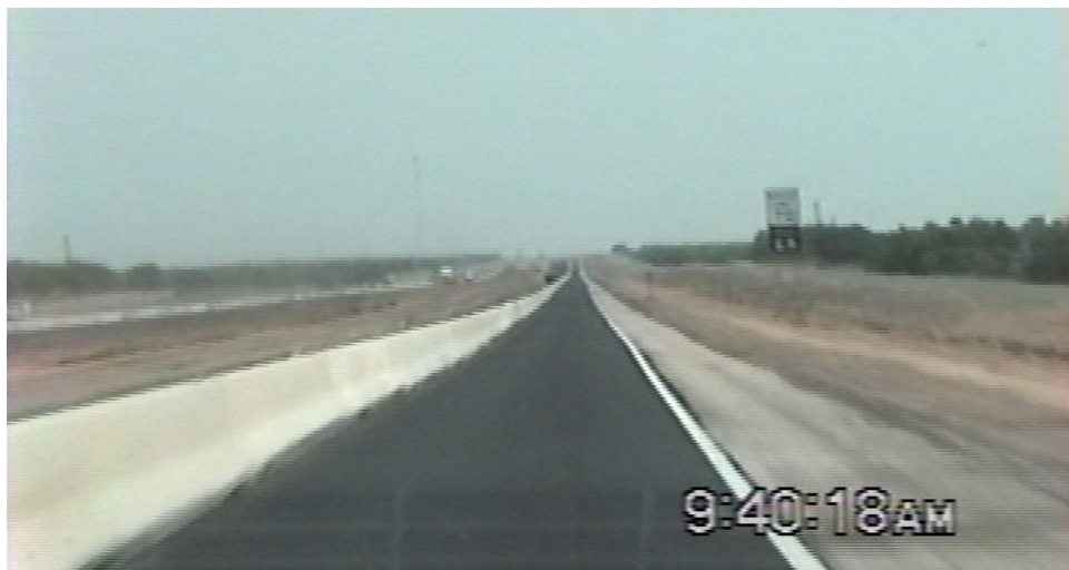
Figure 3-13. Site 3 Photo of Construction Zone.
