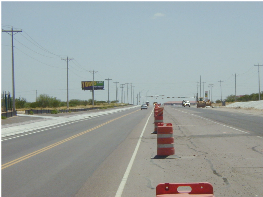
Figure 3-19. Loop 20 Work Zone Approaching Del Mar Boulevard.
