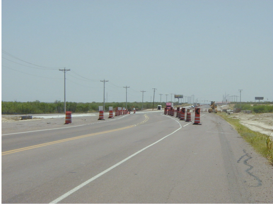
Figure 3-18. Loop 20 ‘S’ Curve in the Work Zone.
