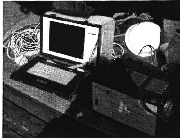
Figure C-2. Traffic Management System Computer.
