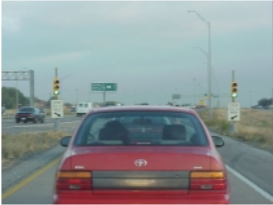
Figure 2. Single-Lane Meter.
