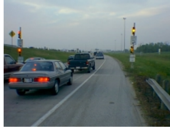
Figure 3. Dual-Lane Meter.
