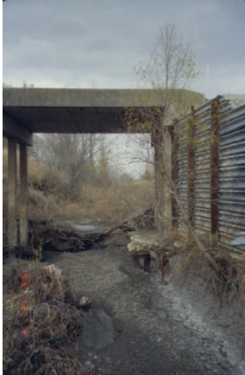
Figure 11.22. Guardrail Wall for Abutment Protection.
