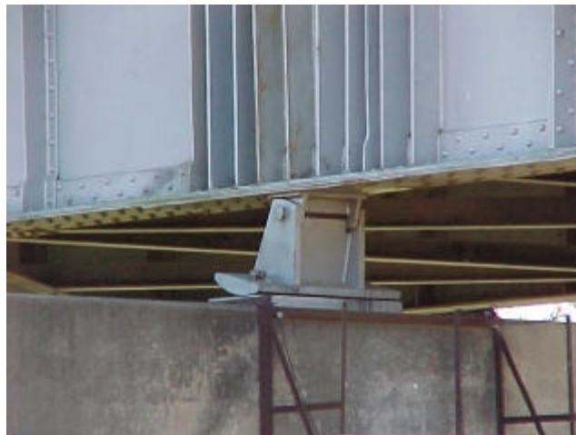
Figure 11.4. Pier No. 50 on the West Bank of the Brazos River.
