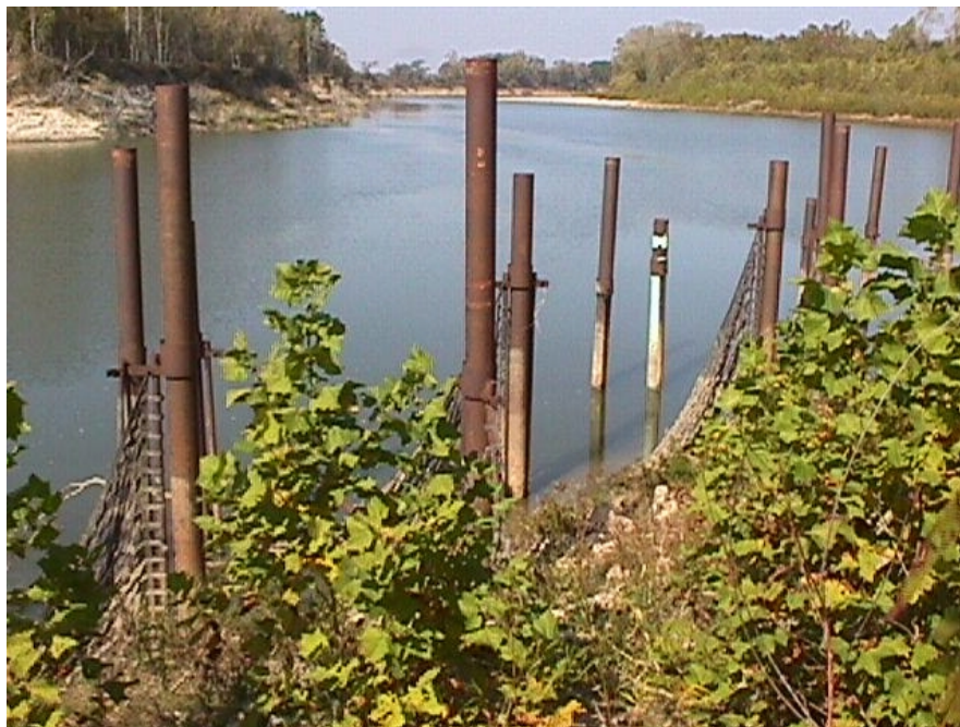
Figure 11.14. Erconet Palisades as Countermeasures.
