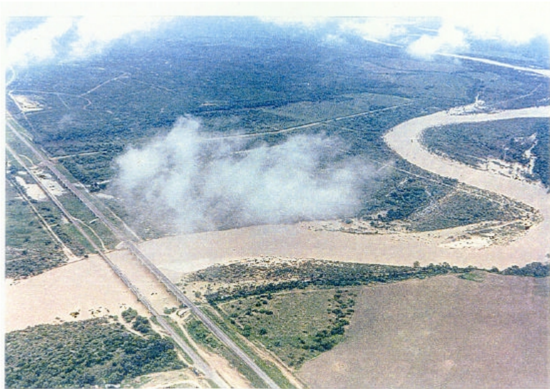
Figure 11.8. U.S. 90 Bridge at the Nueces River –Looking Northwest.
