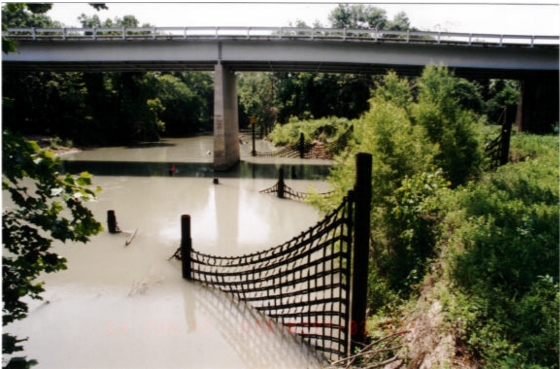
Figure 11.30. Bank of Meander after Installation of Ercon Nets.
