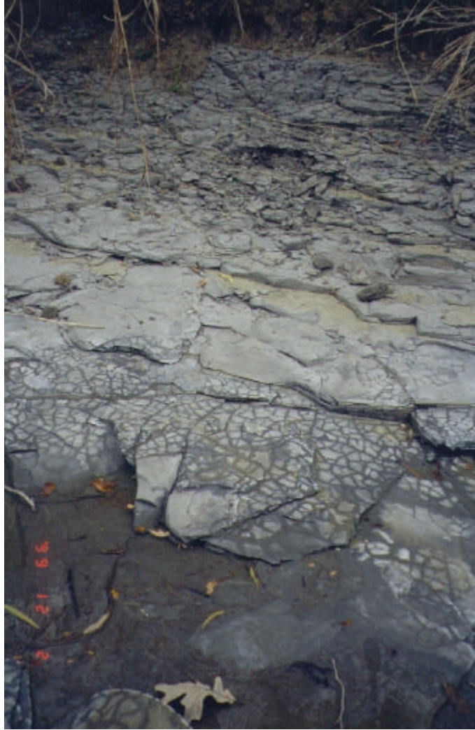
Figure 11.21. Erosion of Clay Shale.
