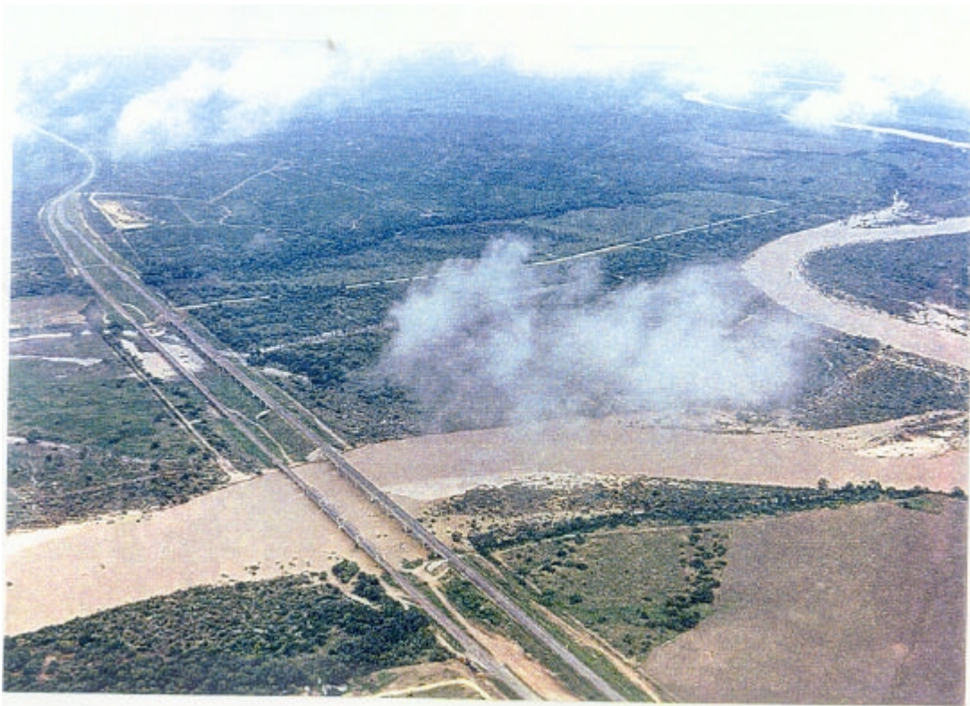
Figure 11.6. U.S. 90 Bridge and Relief Structure at the Nueces River.
