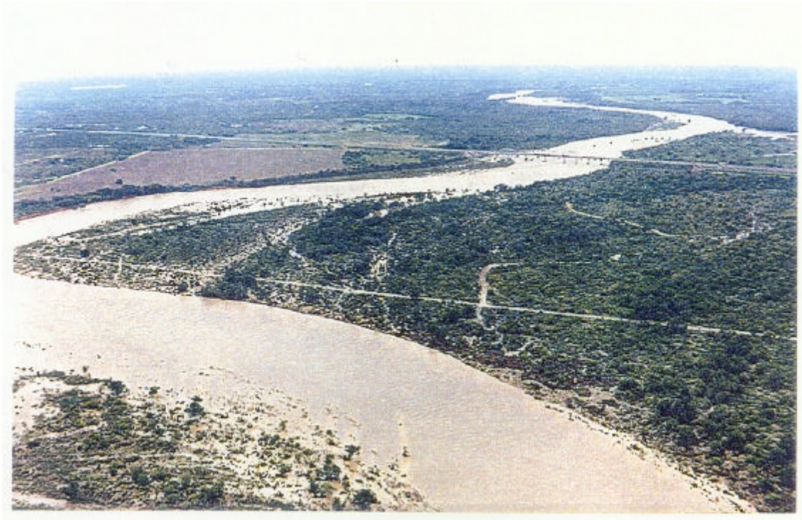
Figure 11.9. Nueces River North of U.S. 90 Bridge (Relief on Right Side)–Looking South.
