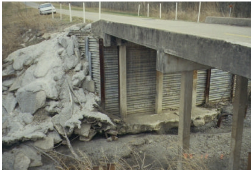
Figure 11.23. Guardrail Wall and Grouted Embankment.
