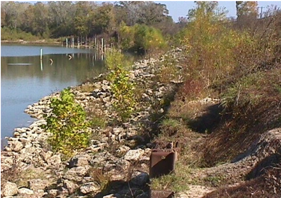
Figure 11.15. Riprap as a Countermeasure.
