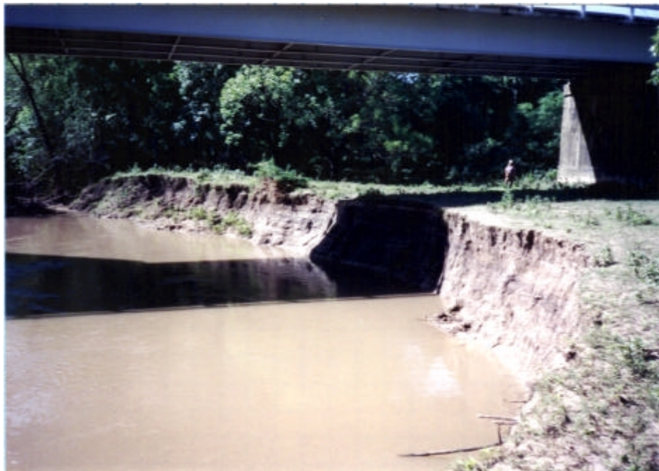
Figure 11.29. Bank of Meander before Installation of Ercon Nets.
